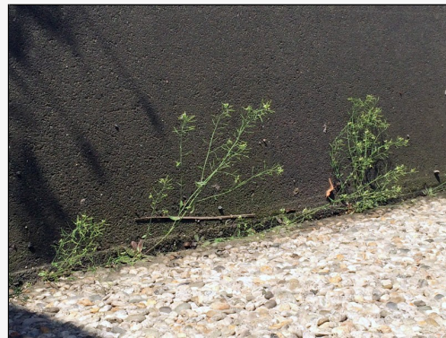
Caption: Base of building wall, Dunedin.
