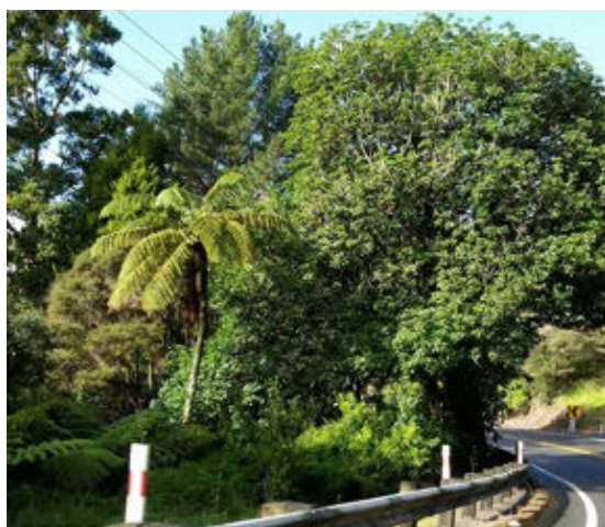
Figure 1. Dome Valley, State Highway 1. June 2015.
